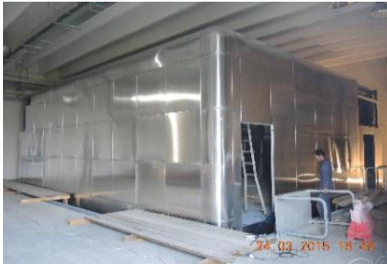
Figure 4.123: High voltage deck hosting all the power supplies and diagnostics dedicated to the plasma source
