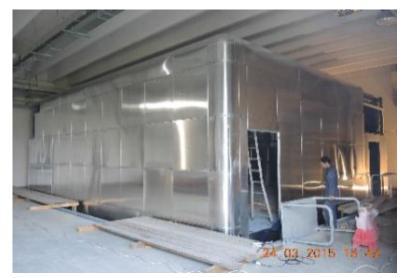
Figure 4.123: High voltage deck hosting all the power supplies and diagnostics dedicated to the plasma source
